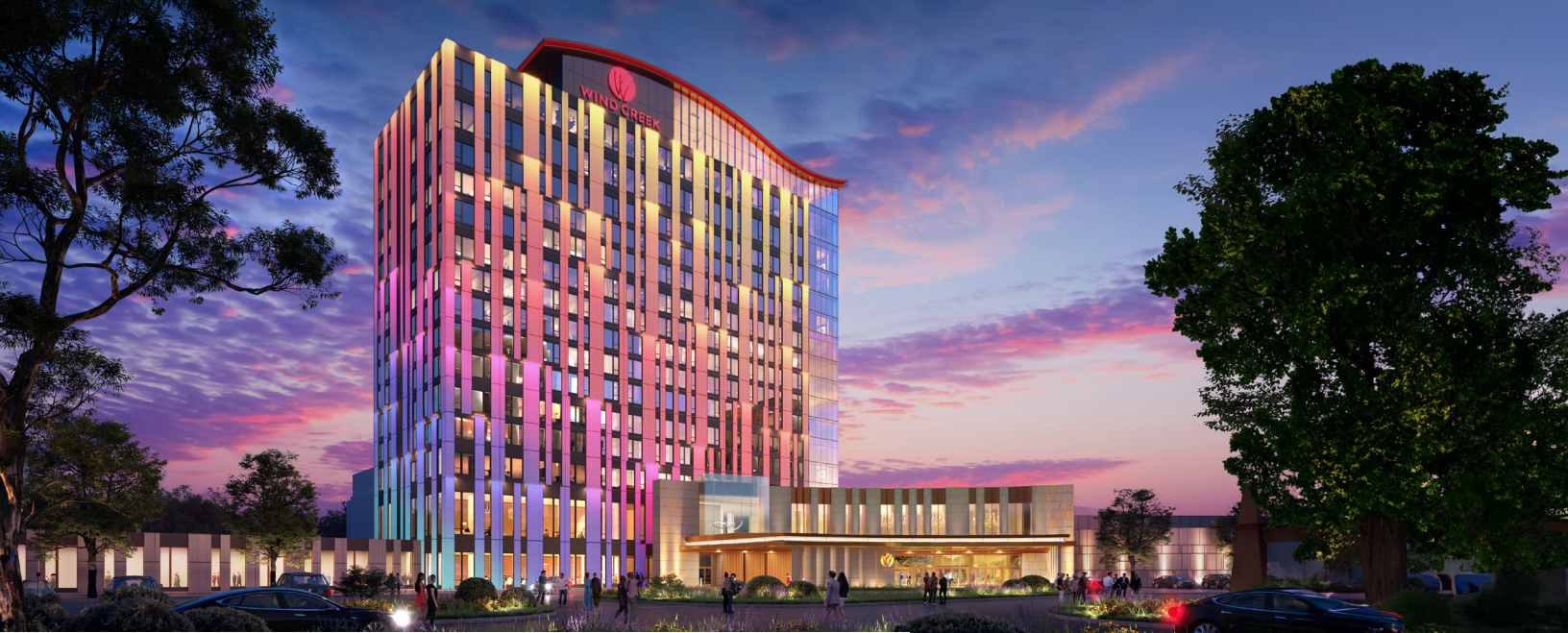
PICTURED Wind Creek Chicago Southland exterior building rendering
