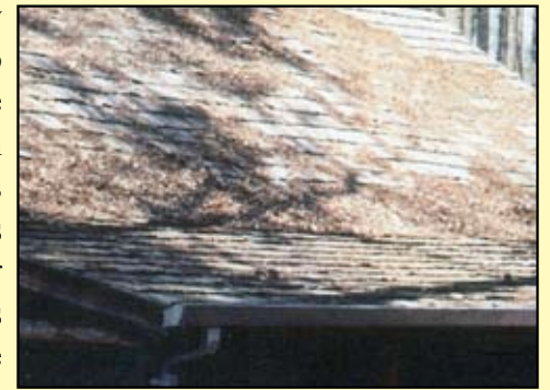
One spark on this roof could be a disaster. Wooden shingles and leaf litter is a hazardous combination.
