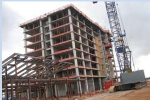
The concrete frame for the 17-story hotel has now reached the 10th floor
