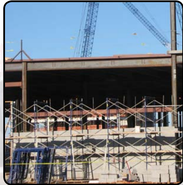
Central Plant and Administration Offices Steel Frame
