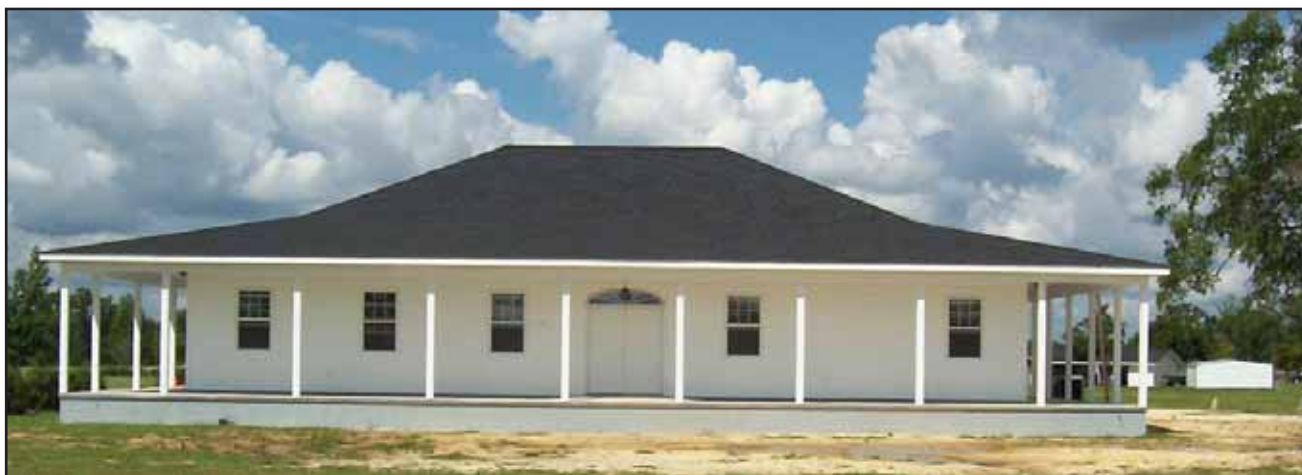
Back of current church - addition just finished
