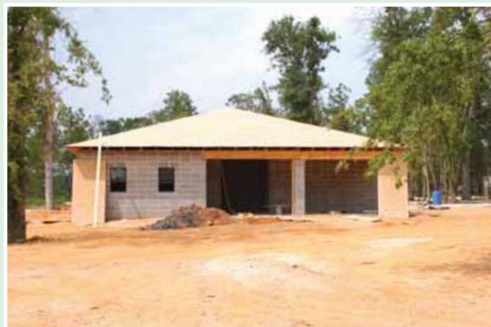
Shower facilities are almost ready
